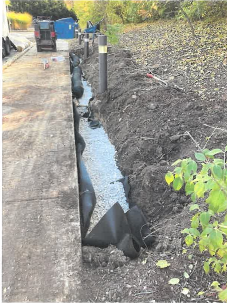
French drain completed
