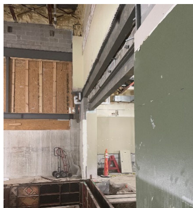
Revised – pushing the elevator shaft over 8”
